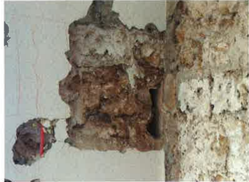
Jaffa Project: damage done by salts soaked from sea and modern cement plasters.
