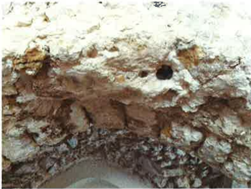
Jaffa Project: damage done by salts soaked from sea and modern cement plasters.
